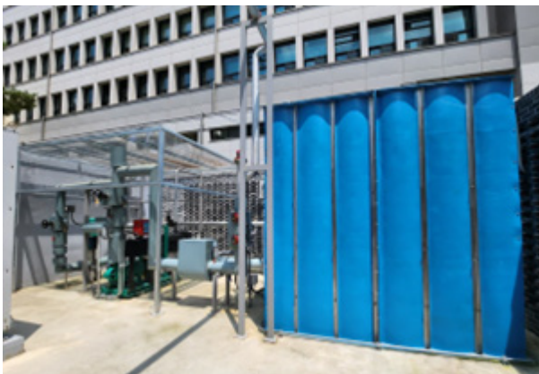
Figure 5: Emergency fire suppression tank and shut-down valve at the Seosomun Hydrogen Charging Station (SMG, 2023a)
